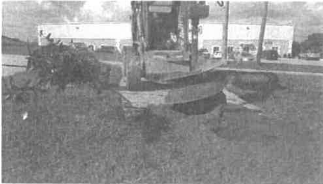
Plywood sheets protect lawn from compaction
