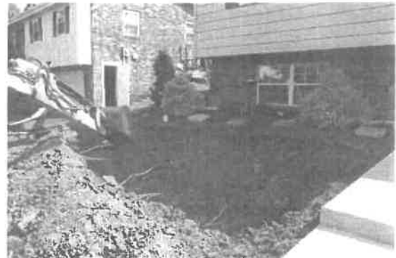
Excavate rain garden at least 10' from foundation
