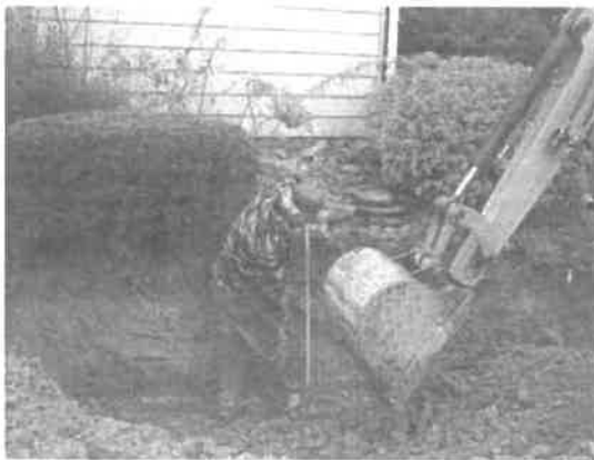
Excavate a drywell at least 10' from foundation
