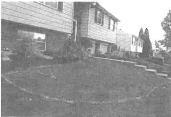
Mark rain garden location to avoid utilities
