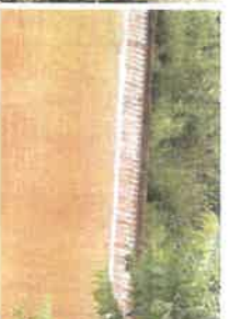
Abandoned mine drainage flows through the treatment ponds.
